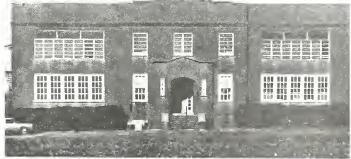
Old Schoolhouse and dormitory
